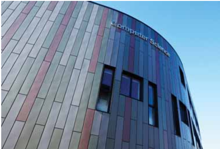
University of York, UK, Designed by BDP, Sheffield, VMZINC Pigmento Red, Pigmento Green and Quartz-zinc Interlocking Panel cladding
