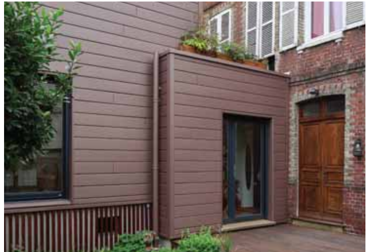
Private House, Ruen, France, Designed by Sarah Bigot, VMZINC Pigmento Red, Pigmento Green and Quartz-zinc Interlocking Panel cladding
