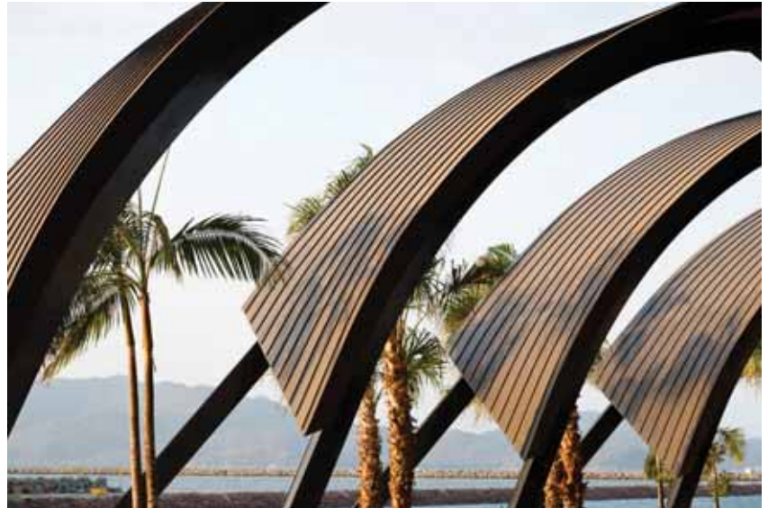
Townsville Cruise Terminal, Designed by Arkhefield Architects, Installed by ZC Technical, VMZINC Athra-zinc Standing Seam, Photography by Angus Martin Photography
